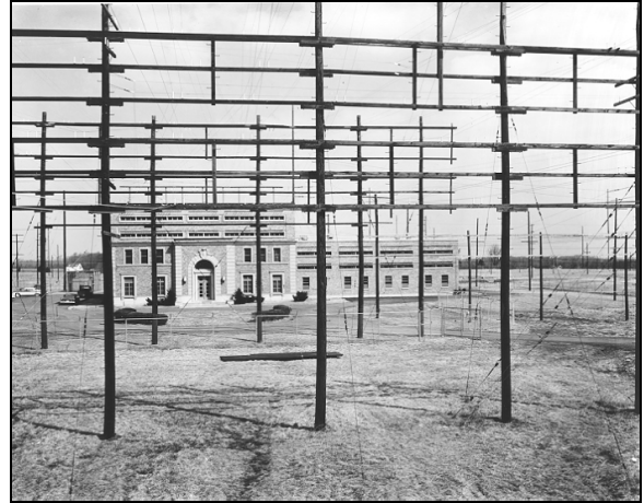
AT&T Main Transmission Building
